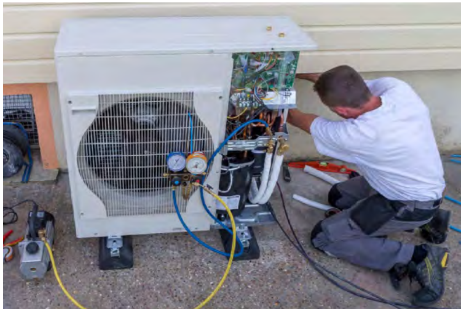
Figure 20 Heat Pump Outdoor Unit Installation in Progress
