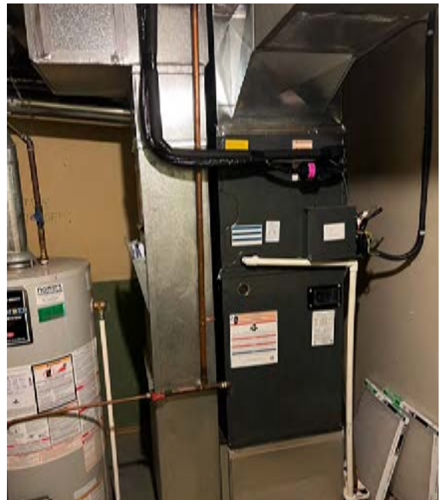
Figure 15 Indoor Unit of a Central Heat Pump
