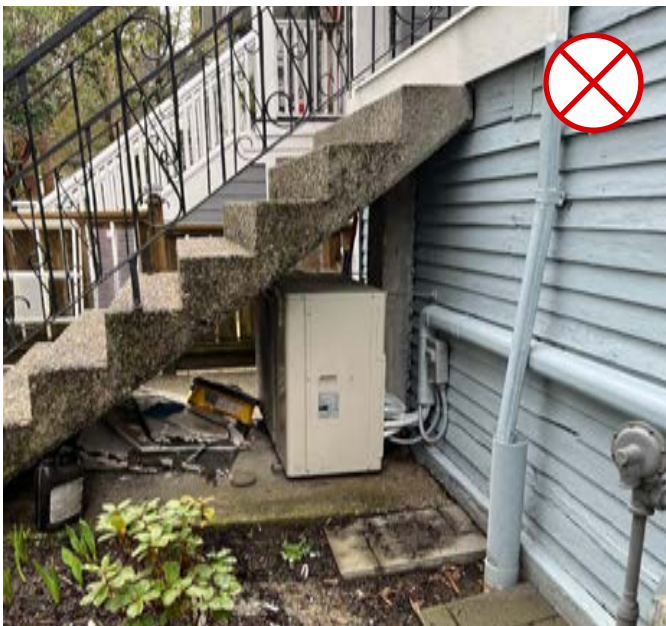
Figure 11 Example of Installation with Inadequate Clearance (left) and Adequate Clearance (right)
