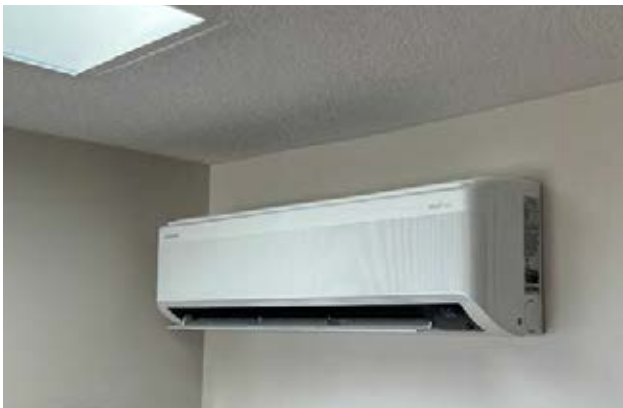
Figure 14 Indoor Unit with Adequate Ceiling Clearance of a Mini-split
